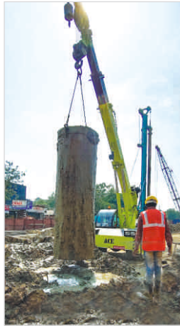
Casing Removal
